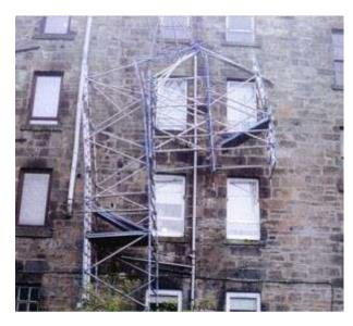
JR Scaffold Services Ltd has been fined after an employee fell eight metres to the ground and sustained severe injuries when the cantilever section of a scaffold he was erecting collapsed.
